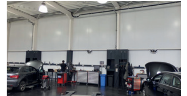
No evidence of fire penetration to interior of the workshop
